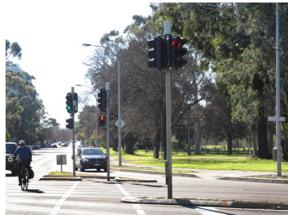
Existing crossing and slip lane on the eastern side of Glen Osmond Road at the intersection with Hutt Road with poor waiting areas and high speed vehicle turning movements
